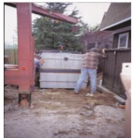
*The seam of this concrete septic tank is sealed with a butyl strip that provides additional assurance that it is watertight. The inlet and outlet have cast in place rubber boots with stainless steel clamps.*
