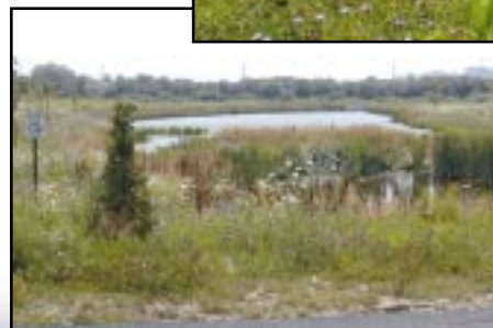
Constructed wetland in the Bailey Brook watershed helps treat runoff from the roads and parking lots.
